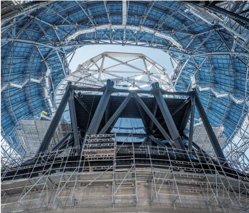
Ponteggio Multicom Extremely Large Telescope (Chile)
